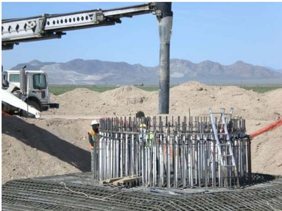
Figure 7.2: Photograph illustrating the construction of the foundation for a wind turbine (photo sourced from www.blm.gov )
